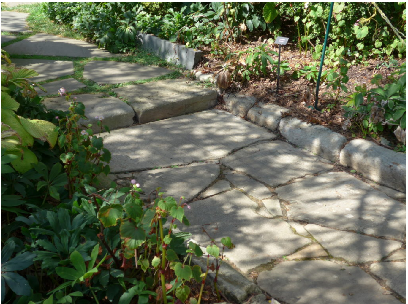
This step will be eliminated to create a small ramp
