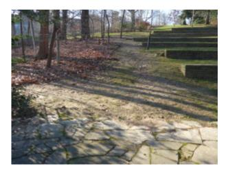
All Hallows Guild is addressing these areas – both because they require amendment and because the Amphitheater has our name on it. We built it and we must repair it. We expect to have the stone floor re-set in concrete to blend with the stonework in the Amphitheater steps, and are investigating measures such as porous paving for the eroded slope. Look at these "before" photographs of the damaged areas and keep watching for "after" pictures as we undertake the work.
