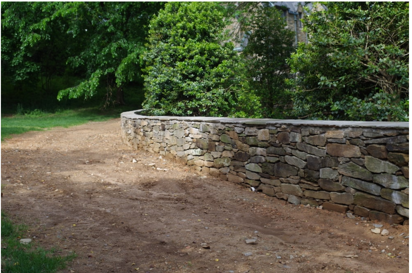
The upper wall of the Nitze Garden, rebuilt Spring 2019
