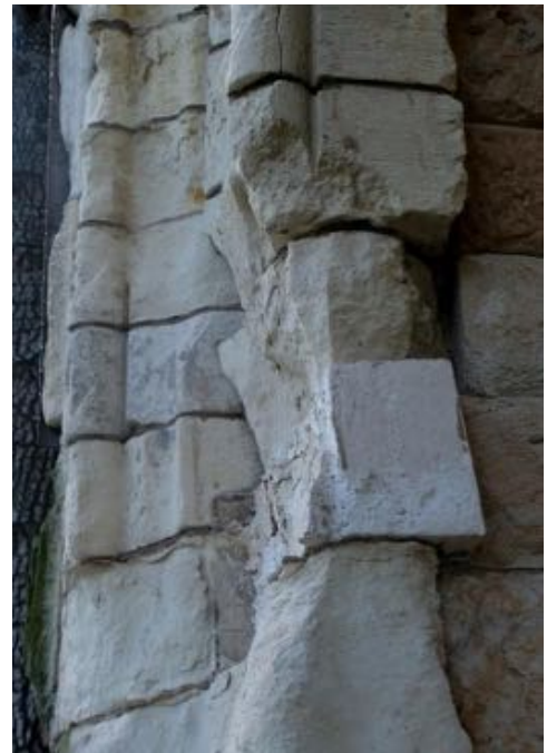
Fig. 3 and 4. Deteriorated blocks of the Norman Arch.
