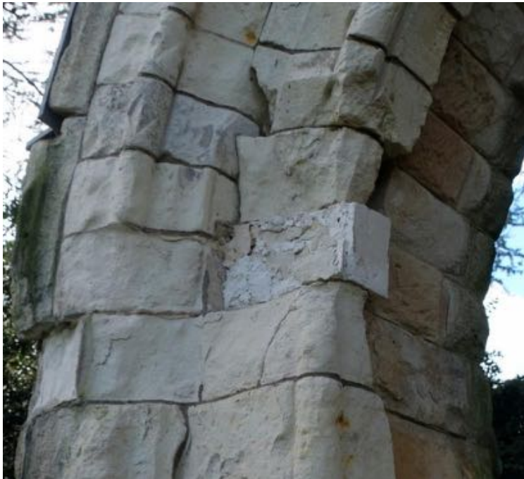
Fig. 3 and 4. Deteriorated blocks of the Norman Arch.
