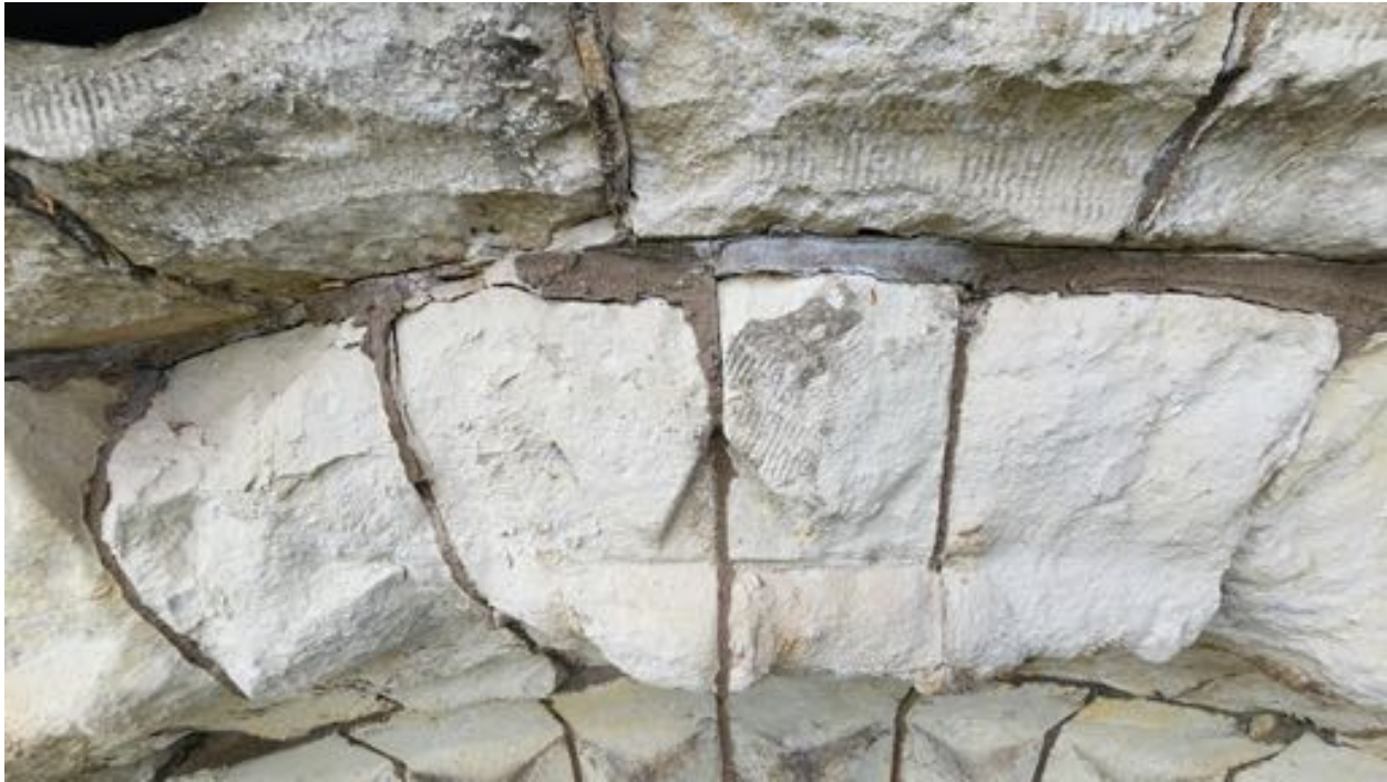
Fig. 5. The fragment of the Norman Arch. Old and extremely hard cementitious pointing mortar before it was removed from the joints of the Arch.
